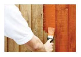
During the drying of alkyd paints several different stages can be identified. The **first process** is the **physical drying** of the paint. In this process, the solvent evaporates and a closed film forms through coalescence of the binder particles. Then **chemical drying** (also called oxidative drying) occurs, a lipid autoxidation process, which means that the paint dries by **oxidation of the binder compound with** molecular **oxygen from the air**.
